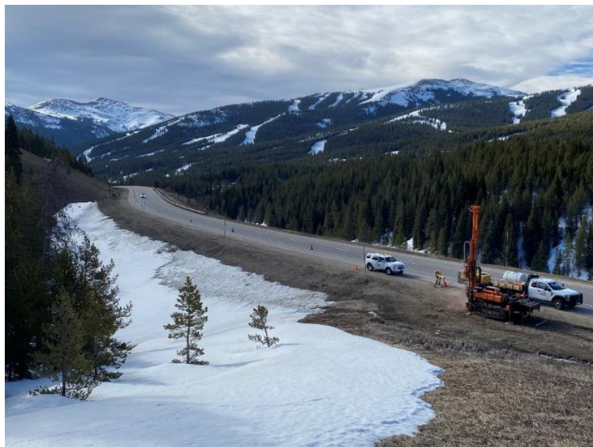
Figure 3. Area 2, Boring B-2 near existing drainage, looking southeast.
